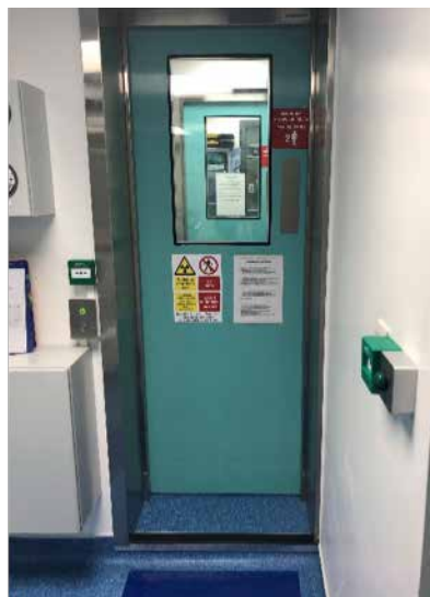
Figure 2: Typical entrance to a radiopharmacy clean room: the clean room door is without a handle, a sticky mat is placed on the floor to remove dust from shoes, there is an interlock at the door, access to the room is restricted, and a sign on the door indicates that this is a radiation control area and shows contact details for the radiation protection supervisor
